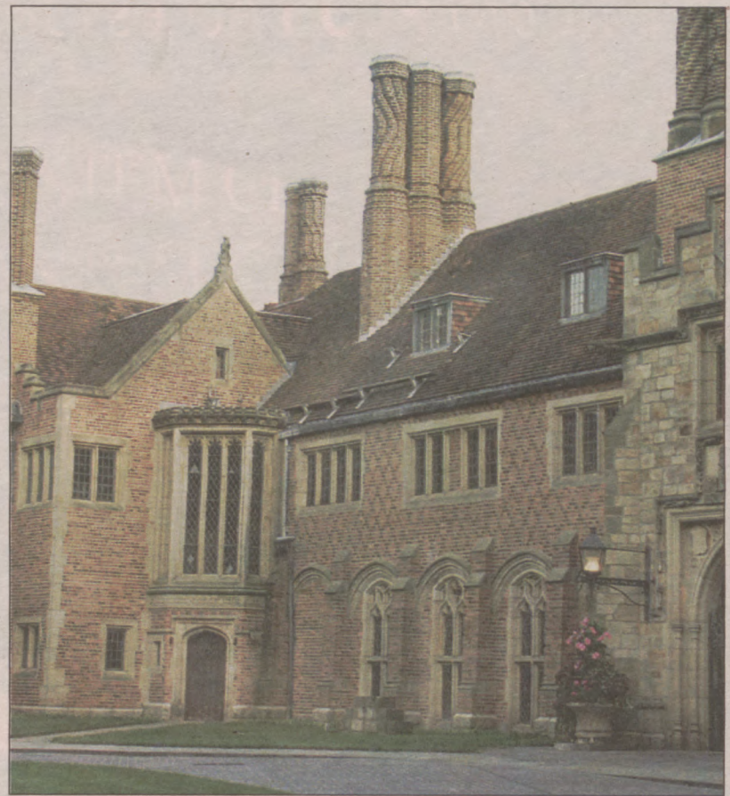
The Oakland Post/DAN WILKINSON Meadow Brook Hall, an 80,000-square-foot mansion built in the Tudor revival style, was home of Matilda Wilson and her family.
