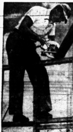
NEW TOOL—A portable electric saw is one of the first items of power equipment on the average handyman's list. The homeshop saw being used here to cut framing members for a new addition to the home can be attached to the saw bench in the workshop as a stationary tool.
