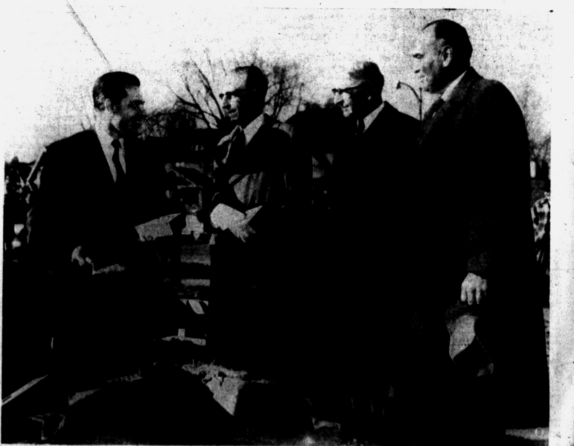
BUILDING STARTED — Congressman William S. Broomfield (R-Royal Oak) and Acting Postmaster Leslie H. Dean Sr. (left to right) add several bricks onto the now under construction $850,000 post office expected to be ready this spring. Retired Congressman George A. Dondero (R-Royal Oak) standing next to Dean and Walter K. Willman, city manager, were also present at the official post office groundbreaking ceremony yesterday afternoon.
