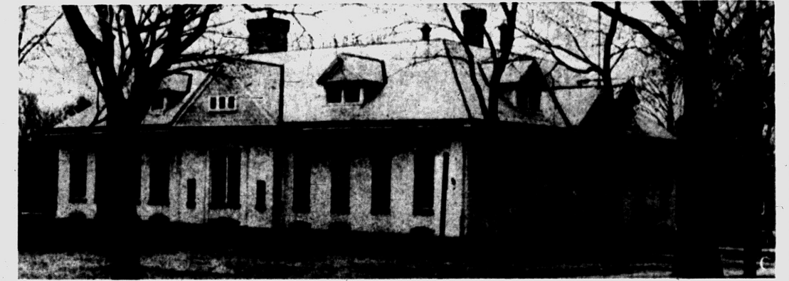
TO BE RAZED—Teachers and students moved out of the Cora C. Bailey School this week. Pontiac Board of Education members have made plans for the 66-year-old building to be torn
