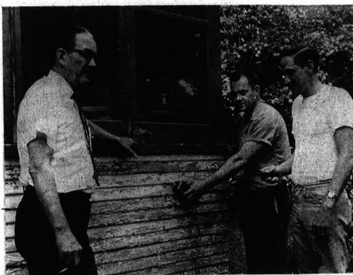
PAINT-UP PROJECT BEGINS — Three neighbors of Mrs. Rose Troiber of 602 Collier begin painting her house. From left are Bert Henson, Ben Fischer and Robert Hoskins. The project was undertaken in conjunction with a citywide cleanup, paint-up, fix-up campaign. This week is Beautification Week and residents have been urged to plant greenery and shrubbery to uplift appearances of their neighborhoods.
