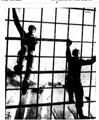
POWER SETUP — Workers scale steel rods which will be part of the Manicouagan Dam face. Dam being built in Quebec wilderness is scheduled to be completed in 1971.
