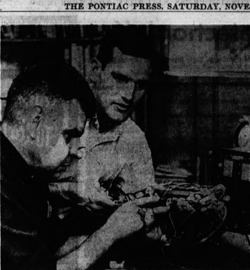
RADAR FOR THE BLIND — Dr. Thomas A. Benham (left), a physics professor at Haverford College, works on the electronic cane he hopes will help the blind. Dr. Benham, blind since 2, works with Don Meeks Jr., a technician with a firm that may develop the device. The cane is intended to carry radar and tell the carrier how far away objects are and in what direction.
