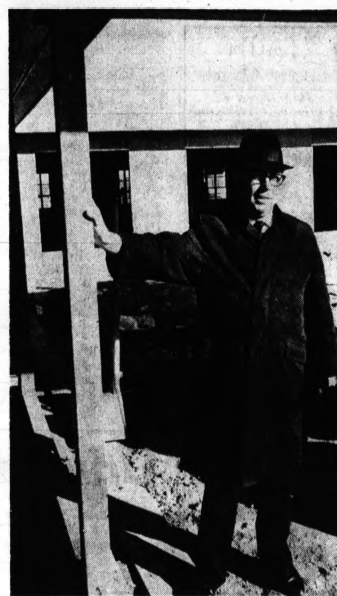
CHECKS CONSTRUCTION —Looking over the construction of the new Church of God going up on Walton Boulevard just east of Joslyn is the Rev. Cheslie N. Collins, pastor. The congregation is presently worshipping in the church at 575 E. Pike.
