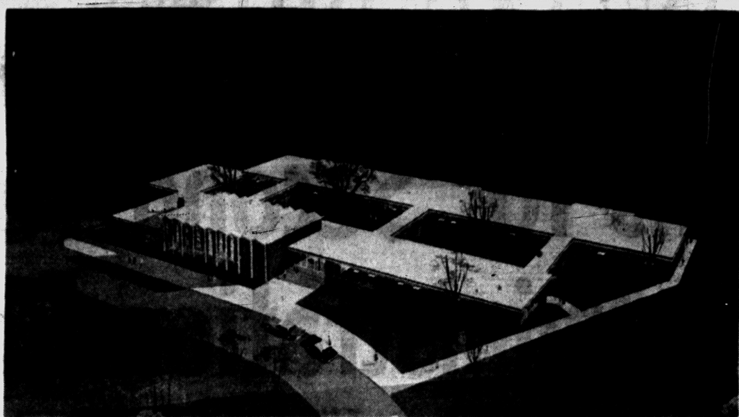
COURTYARD SCHOOL —Hickory Grove school district in Bloomfield Township will have this school completed by next fall, officials plan. In each of the three courtyards, a hickory tree will be growing, in view of the nine classrooms, library, and offices. Under the saw-
