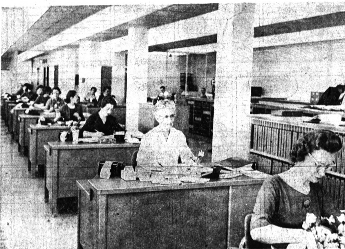
CONDUCTIVE TO EFFICIENCY — Workers in the new county treasurer's office are provided plenty of light by alternate rows of fluorescent lighting that run the length of the new wing. Rows of windows on the opposite wall from the one shown
