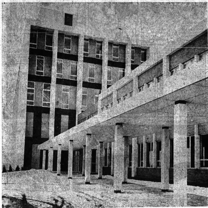
MODERN CLASSIC —The use of strong geometrical designs in modern architecture is evidenced in the new county courthouse and west wing. Here, marble columns line the walk in
