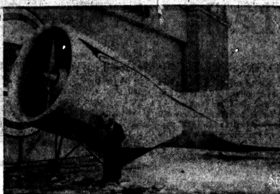
LOOK MA, NO WINGS! — Full-scale model of a wingless airplane is shown in Cedar Rapids, Iowa, with its designer, Dr. Alexander Lippisch. The Army-Navy developed "Aerodyne" can take off and land vertically and fly normally. Two contra-rotating propellers force air through the fuselage and out controllable vents in the belly. Cockpit will be located aft under a canopy in the vertical stabilizer.
