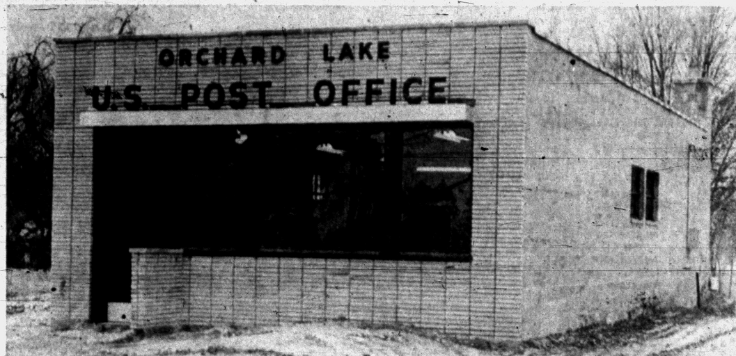
ORCHARD LAKE POST OFFICE TO OPEN — The new Orchard Lake Post Office on 3735 Commerce Rd. will be open for business on Monday morning at 8 a. m. Postmaster Hawkes plans to have two
