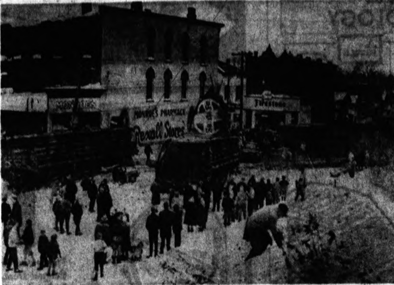
TRAIN DERAILS — Spectators survey the wreckage after 15 cars of a New York Central freight train plunged off an overpass into downtown Dunkirk, N.Y. Three automobiles were demolished and several buildings damaged.
