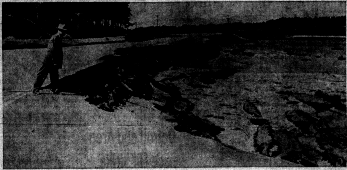
QUAKE TAKES OUT ROAD —About 1,000 feet of this main road along Lake Merced in the western part of San Francisco was broken off by the force of Friday afternoon's earthquake and sent tumbling into the lake. The damage shows the intensity of the tremor.
