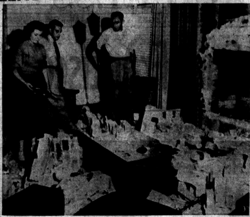
WHAT A MESS!—Mr. and Mrs. Louis Martinelli and neighbor, Joe Scafidi, center survey damage done to the living room fireplace of the
