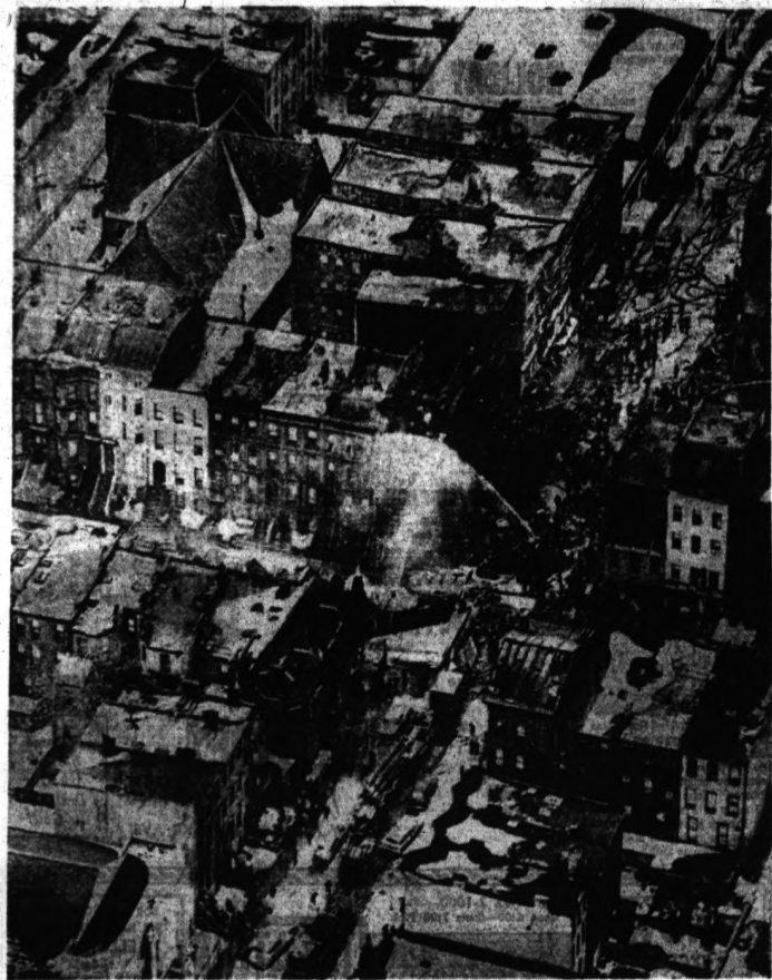
WHERE DISASTER STRUCK —This was the scene in Brooklyn Friday as firemen played streams of water on one of the buildings set afire by the crash of a United Airlines jetliner following a collision with a TWA airliner over the New York area. It is almost miraculous that the plane fell into an intersection of the
