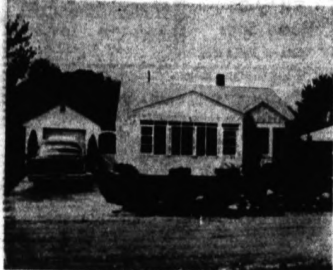
THREE YEARS AGO — This is the Clem Snarrs house as it was when the Snarrs moved here from Detroit five years ago. When they enlarged this 28x32 home, they built over and around the original structure. The former living room is now a bedroom; the garage is a recreation room.
