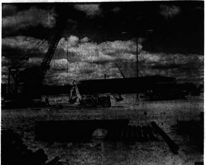
MOTT HIGH PROGRESS — Workers are busy at the 76-acre site at Pontiac Lake Road and Scott Lake Road in Waterford Township where Mott High School is scheduled to open in the middle of the school year. Final completion date
