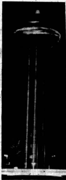
UNIQUE TOWER — Night view shows 250,000-gallon, 140-foot stainless steel-clad water tower at the General Motors Technical Center at 12-Mile and Mound Rds.
