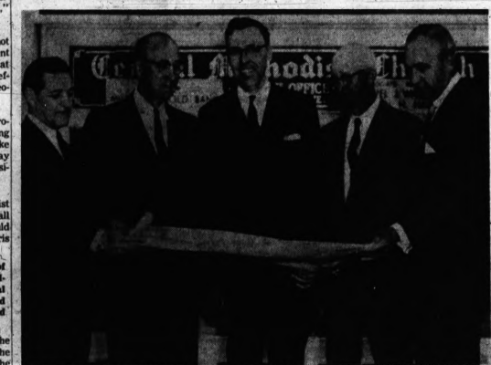
COMPLETING SALE — Representatives of Central Methodist Church in front of the new building. From left are: William H. Taylor Jr., president of the church; Elbert M. Witold, chairman of the church building committee; Dr. Milton H. Bank, pastor; Howard Simmons, chairman of the church's official board; and Bruce J. Arnett, realtor.
