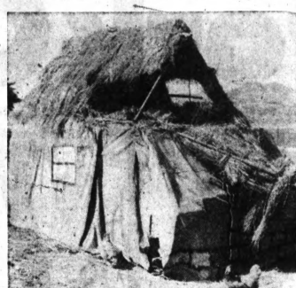
FOOLS' DEN — Little grass-thatched shack in a Korean village is a camouflage project of the U.S. 1st Cavalry Division. "Shack" is shown with portion of roof lowered to permit clear field of fire for a turret-mounted 50-caliber weapon.
