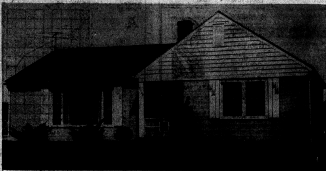
IN CHEROKEE HILLS — The first of the three houses built by the brothers, this 44-foot long cement block home is painted pink. Trim is white. Note the initials on the shutters. Six months after the basement was dug, the Ward Newmans moved in even though the house was not done. There are four girls in the family: Ruth Ann, 16; Sandra, 11; Jacklyn, 5; and Brenda, 3.
