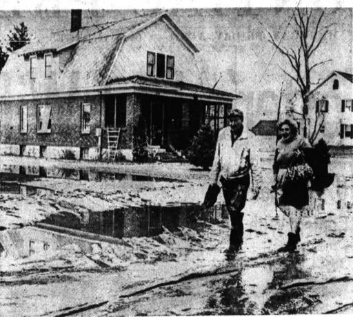
BIG TASK AHEAD —Mr. and Mrs. E. L. Reynolds walk through deep mud and water after making an inspection trip to their Chaska, Minn., home (left), yesterday. They did some cleaning but were hampered because there was no water, gas, electricity or heat. The high-water mark can be seen on the side of this house halfway up on the main floor windows.
