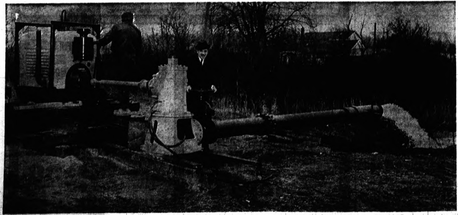
PUMPING TEST — Walled Lake City Manager Royce Downey tests the new water pump being installed, which can handle up to 6 million gallons a day. The $2.2-million system should be in operation within two months. The well is reportedly
