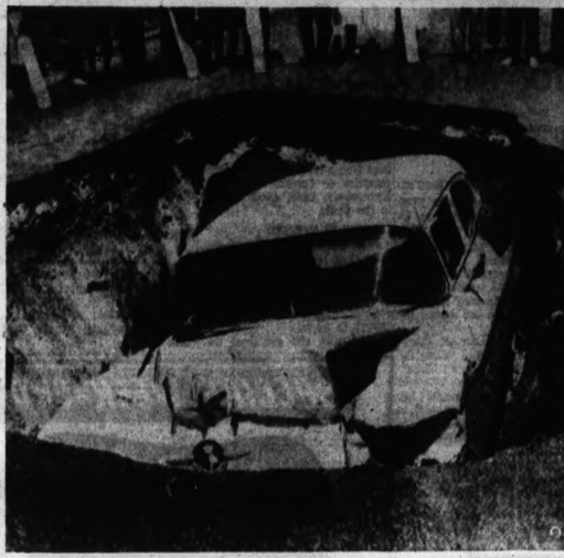
HOLED UP — The bottom dropped out of whatever plans Richard W. Tawak of Chicago had for the rest of the day when he found himself looking up at the pavement. The street gave way suddenly smashing his car and sending Tawak to the hospital to be treated for shock. A leaking main sewer had washed the earth away from beneath the pavement.
