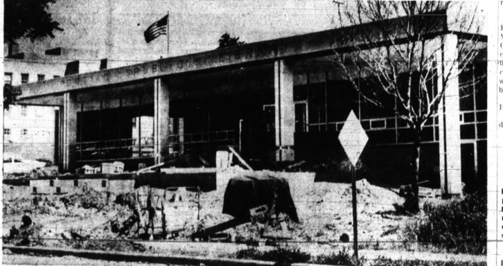
NEARING COMPLETION — Construction of the $500,000 Pontiac Public Library building should be finished in about a month. Bundy Construction Co., the general contractor, said the exterior
