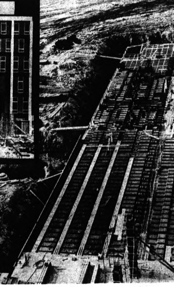
ON SCHEDULE — Good weather has aided workmen of the Bundy Construction Co. of Pontiac in building the west administrative wing of the new Oakland County Courthouse. The basement of the new addition has just been completed and the first floor of the three-story structure is now being erected. The first completed section of the administrative wing is pictured here in a view from the Courthouse and the inset shows it in relation to the lower unit. The 50-by-284-foot addition will house offices now in the Oakland County Office Building, 1 Lafayette St.
