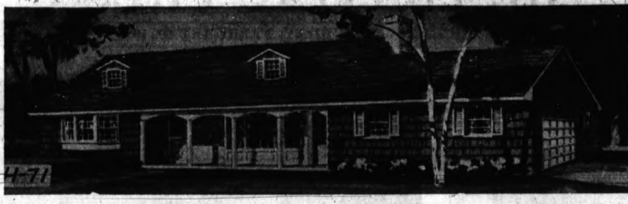
HOSPITABLE EXTERIOR — There's a welcoming air to the traditional design and materials of this 1½-story expansion house, which has 1,662 square feet of living area on the main floor and 964 additional square feet of habitable space above.
