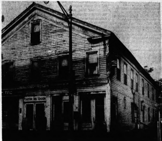
TO BE RAZED — The old Rochester Hotel on the southwest corner of Main Street and West University Drive, Rochester, will be torn down this spring. A longtime "eyesore" of the community, the old hotel has been termed a fire hazard and dangerous to public safety by local building, electrical, fire and health officers. Now it only houses a television and radio repair shop plus a bus line waiting room.
