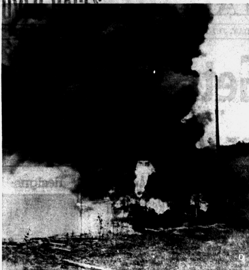
BILLING SMOKE —Smoke rising from a blaze which destroyed three old buildings used to store surplus paint from wartime operations churned over Avon Township yesterday afternoon, drawing many residents to the scene. Formerly owned by the Alcoa Manufacturing Co., the property was currently owned by Fred Weine, Jack Young and V. J. McEvoy. Rochester Fire Chief George Ross estimated the damage at $5,000. No one was injured. The cause has not been determined.
