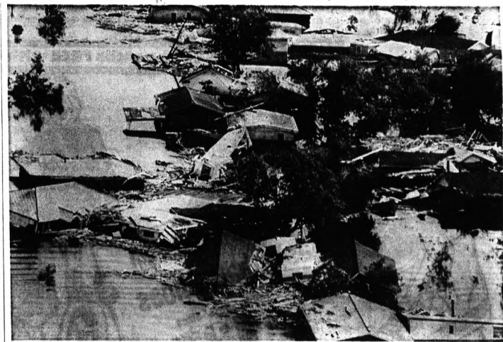
BATTERED BURAS —This was once the town of Buras, La., some 30 miles southeast of New Orleans on the Mississippi River. Hurricane Camille ripped through the town
