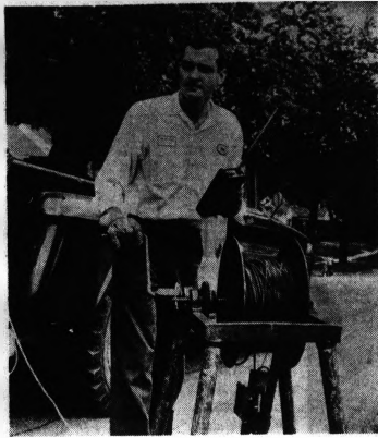
TOUGH PULL —This Oakland County DPW construction inspector is actually pulling a television camera through a sewer every time he turns the crank. Robert B. Winter was part of a team which used TV cameras to scan the inside of the sewer system for defects and illegal connections.
