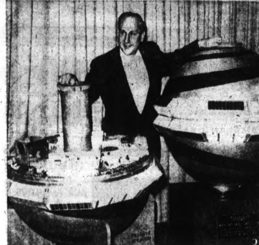
"OUR NEW BABY" — Laying proud hands on the new U. S. Transit IB navigational satellite is Dr. R. B. Kershner of the Johns Hopkins University applied physics laboratory. He explains at a Pentagon news conference that the satellite could provide a ship with a fix on its position with no more than a half-mile error. The new moon, launched Wednesday, was the third satellite the U. S. has lofted into orbit in the last 33 days.
