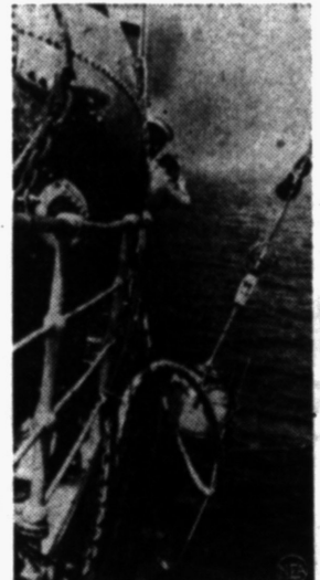
Dropping buoy to mark end of cable near the shore. Buoys make work easier if final splices have to be made at night.
