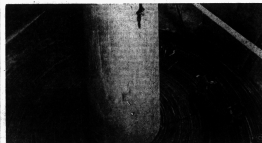
Loading cable in the tanks of H.M.S. Monarch. This operation often takes weeks, but the care taken pays off in that the ship cannot afford tangles or breaks when under way. The 1950-
