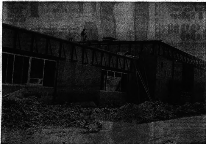
FINISHING TOUCH — Workmen have been putting about 85 tons of a gypsum concrete roof on the additions to the former West Bloomfield Junior High. The building will be used as the high school this fall.
