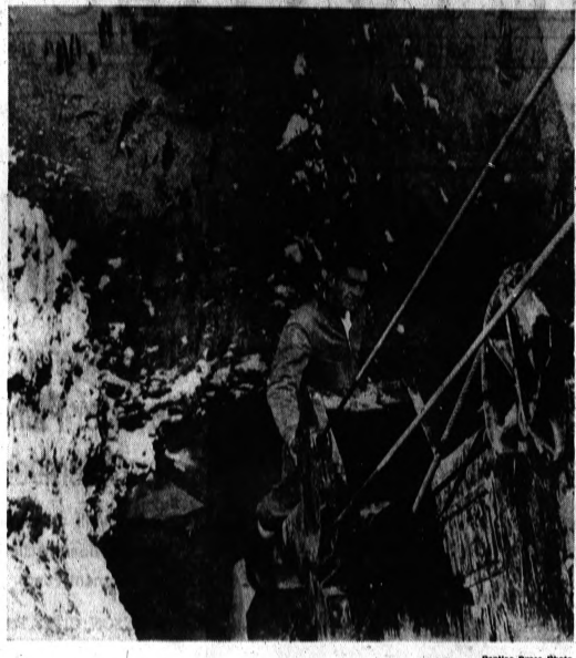
LEAKY PIPE—County Courthouse maintenance men have been working to repair a broken water main into the building since last Wednesday. Andy Vascaseno, 4265 Meyers, Waterford Township, is seen standing near the bottom of an 18-foot hole where the break finally was located. Workmen expected to have the 8-inch water main repaired by tomorrow. Meanwhile, water is being supplied into the building by a temporary hookup.
