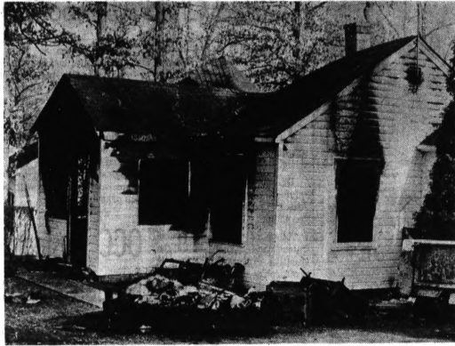
FATAL FIRE—Fire swept through this home in Pontiac Township early today and killed one man, Horace Akerley. Cause of the blaze, which gutted the house, is still under investigation.
