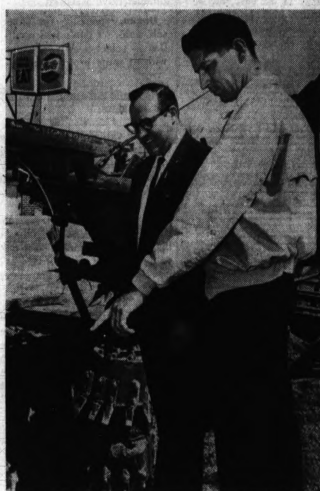
WATER PROJECT STARTS — Waterford Township's $1.5-million water project to interconnect the existing 10 sewer systems got under way yesterday. Township Supervisor James E. Seeler (left) and Kenneth Squiers, water department superintendent, were on hand as main-laying began on M59 at Crescent Lake Road. A total of 135 miles of water mains will be laid.
