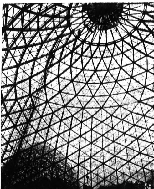
TIP TOPPING — Workman waits near top of a Mitchell Park Horticultural Conservatory structure in Milwaukee, Wis., as crane lifts one of final forms for placement.
