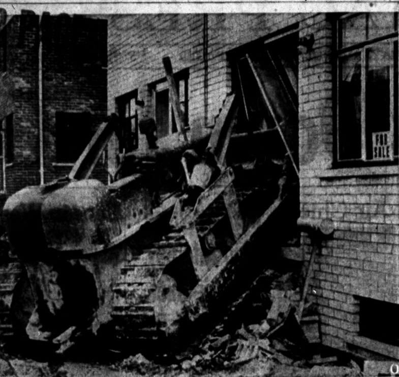
UNEXPECTED VISITOR —Without so much as knocking, a visitor got into the Harry Woody home at 543 Granada this morning. According to witnesses, the operator of a bulldozer struck a utility pole while leveling earth in the new subdivision where the house is located. When sparks started showering about him, the driver leaped off the still-moving machine, which continued rumbling right through the Woody back door. No one was home at the time.
