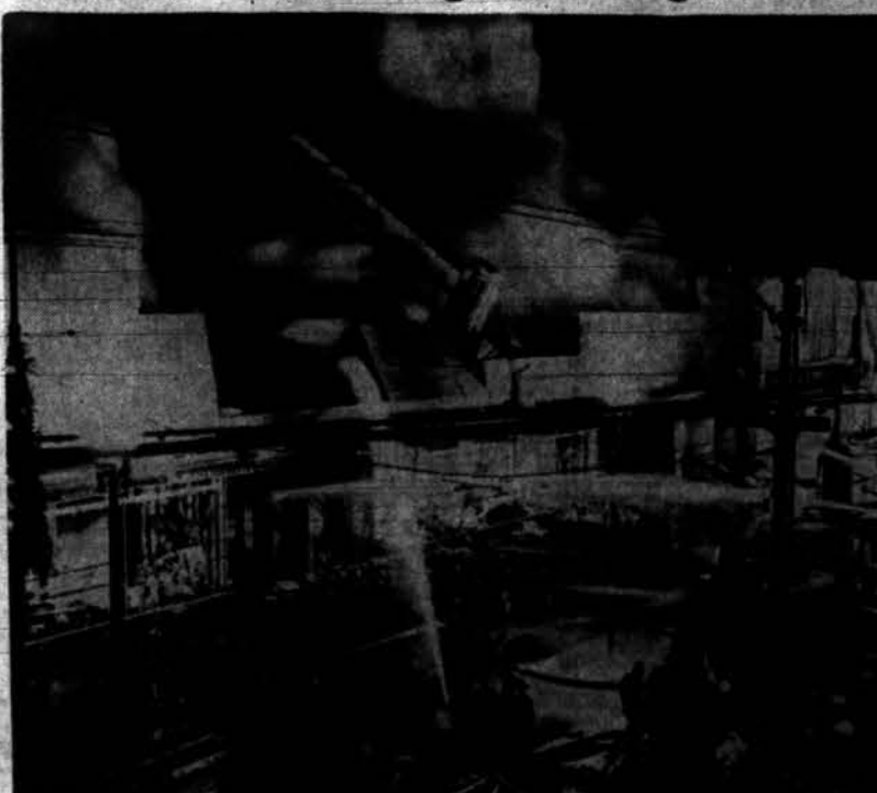
MILLION-DOLLAR FIRE — Smoke billows above the Goldblatt Bros. department store in Chicago's northwest side as firemen fight a blaze of undetermined origin which destroyed the struc-
