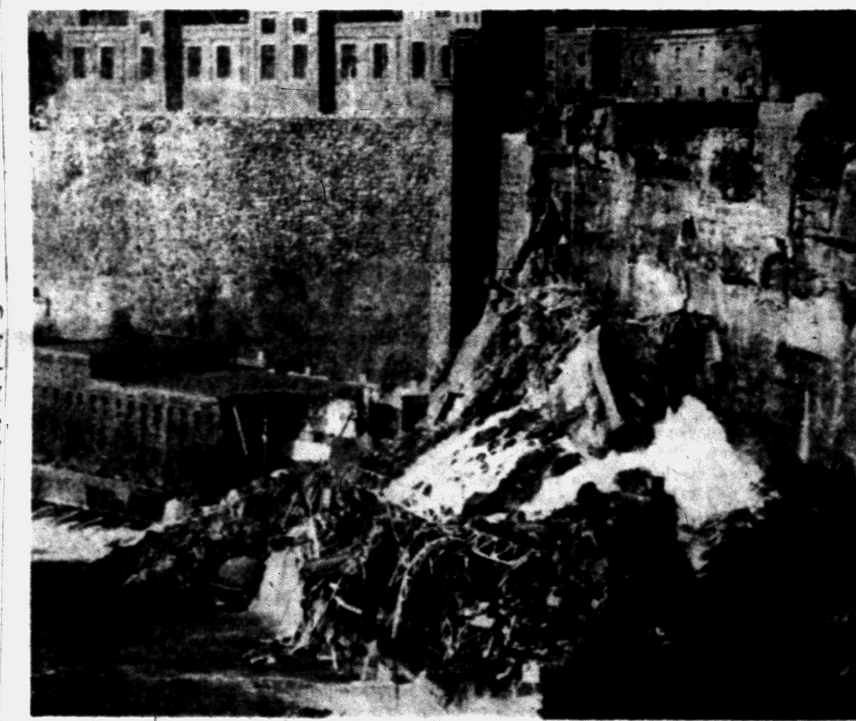
ONE KILLED, 40 ESCAPE — A section of the Niagara Mohawk Power Corporation's Schoellkopf Power Station lies under tons of debris today at the base of the American side of the Niagara River gorge. Picture was taken with a telephoto lens from the nearby Rainbow Bridge. Power station is about half mile below Niagara Falls.
