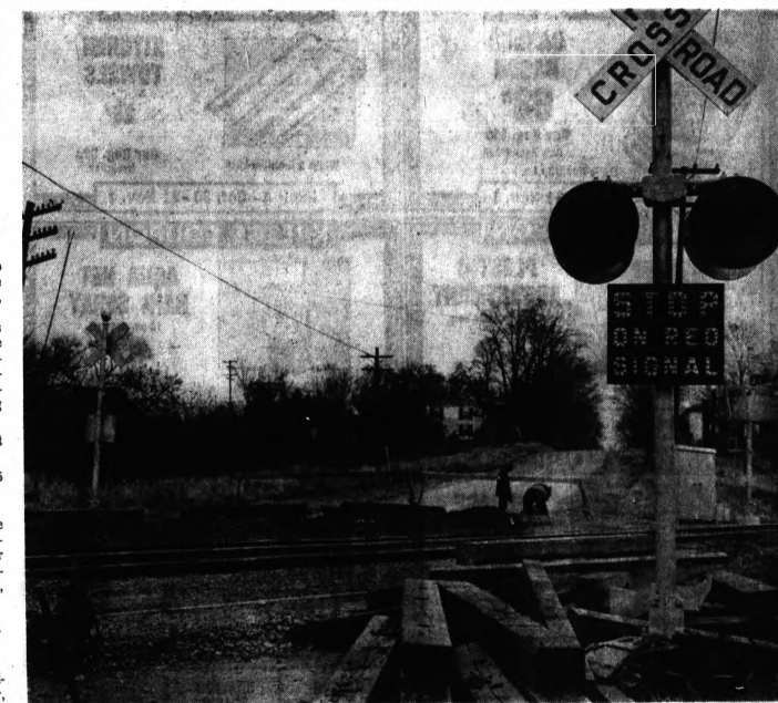
ROAD CLOSED — A grade crossing on Davisburg Road just east of the village is being reconstructed by Grand Trunk Western Railroad maintenance workers. The road was closed last week while the crew worked on the crossing.
