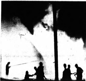
OIL STORAGE TANK HIT Firemen battle the flames as burning oil pours out of a storage tank at the terminal of the American-owned "Tapline" oil pipeline in Sidon, Lebanon, today. The hole and fire were caused by a bazooka rocket, believed to have been fired by Palestinian guerrillas.
