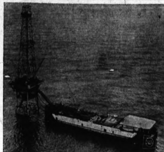
OIL FROM THE OCEAN —Farthest offshore oil drilling installation in this platform 70 miles off Louisiana in the Gulf of Mexico. Built by CATC (a group of four oil companies), it rises 225 feet above the water, which is 180 feet deep at this point. The tender alongside the rig holds the pipe and other drilling gear and provides eating and sleeping quarters for the crew. Platform at aft end is for helicopters.
