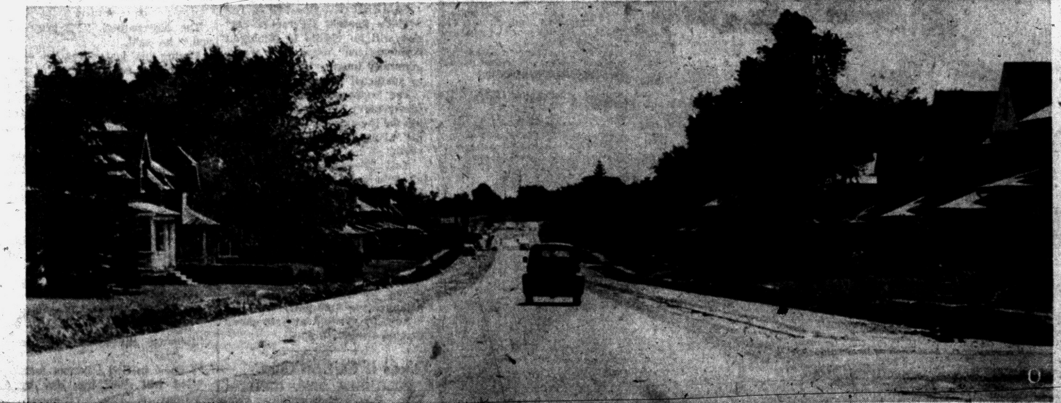
PERRY SHAPING UP — A view of Perry street, looking south from Joslyn, shows most of the concrete paving in but curb and gutter still lacking. The roadway is paved between E. Huron and East Boulevard. The entire 3.9 mile widening
