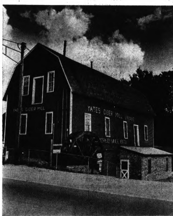
LANDMARK — Yates Cider Mill, built on the Clinton River when it was still a major means of transportation, today still turns out apple cider by means of its water-powered press. There are still a number of apple orchards in the community, although their number is decreasing.
