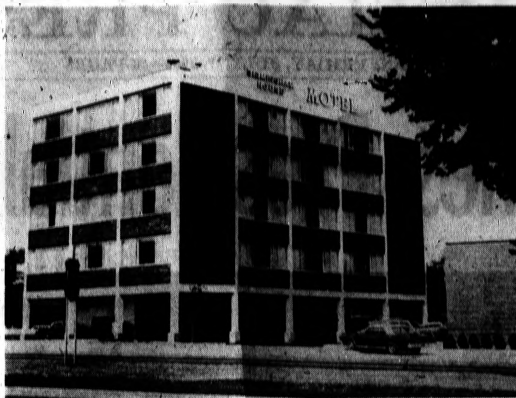
SKY'S THE LIMIT — Birmingham's skyscraper is the new five-story tower of the Birmingham House Hotel. The $500,000 addition to the hotel at 145 S. Hunter increased the total guest capacity to more than 100. The structure also contains meeting and banquet rooms and a coffee shop. Owned by Asher N. Fitch and Stanley I. Aaron, the hotel was established in 1909. The newest addition opened a week ago.
