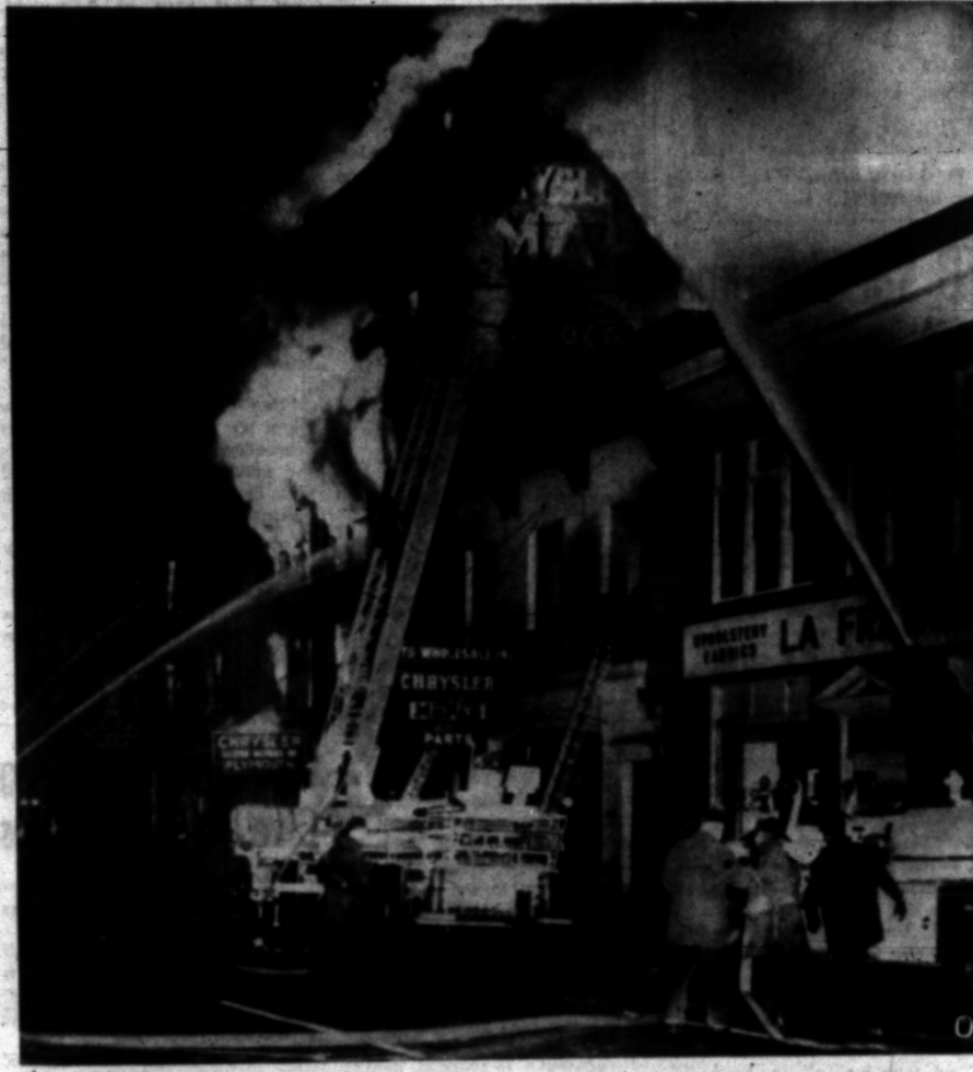
BATTLE 12-ALARM BLAZE—Several hundred new and used cars were destroyed in Baltimore today when a 12-alarm fire swept through three buildings housing the Martin Motor Co. Total damage was estimated at one million dollars. At least 30 persons were evacuated from nearby apartment houses in sub-freezing weather as a precautionary move but were allowed to return to their homes when the blaze was brought under control two and one-half hours after it started at 4 a. m.
