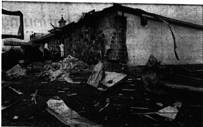
Bedell's Restaurant in Bloomfield Township, Damaged By Bomb
