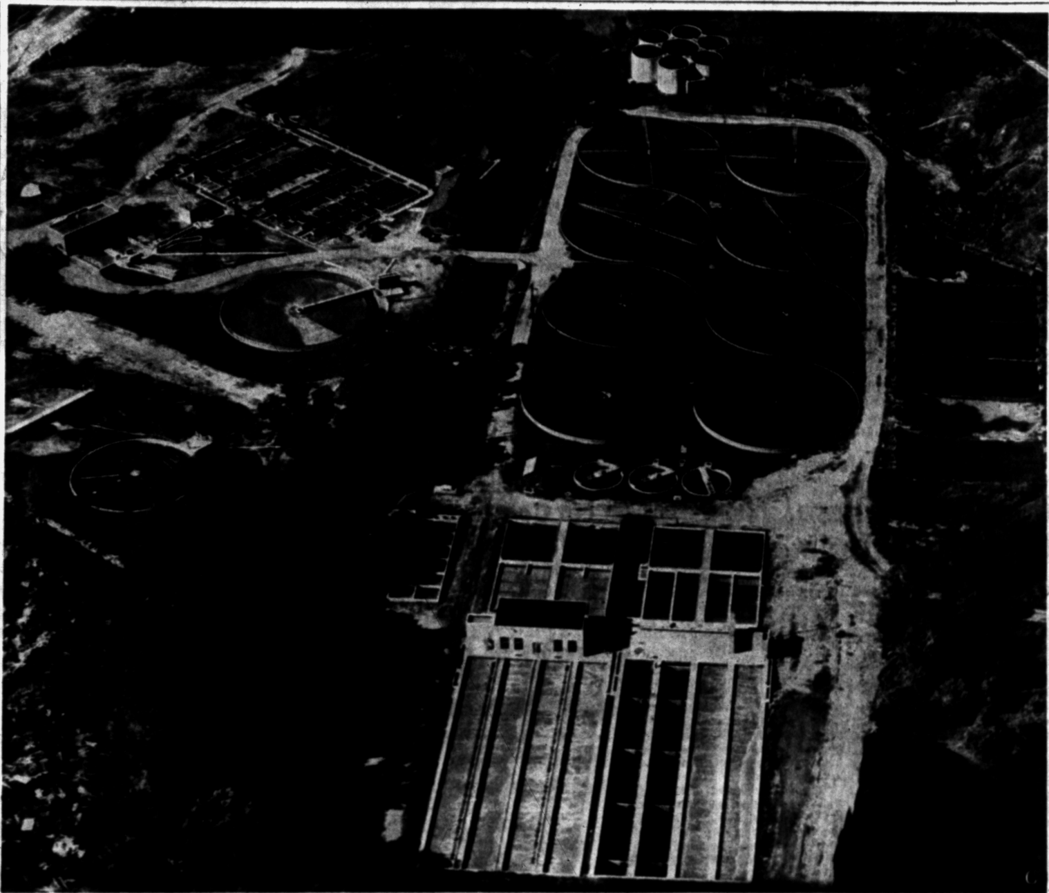
SEWAGE PLANT EXPANSION —Improvements completed this year are shown in this aerial photo of Pontiac's municipal sewage treatment plant at Featherstone Ave. and East Boulevard. The chlorine contact tank (left and below the eight circular trickling filters) had its capacity doubled with an extension of the lower section. Across the Clinton River from the eight filters is a primary sedimentation tank, two years in
