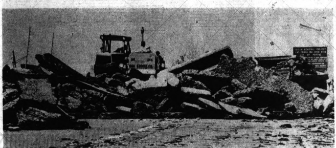
CRUNCH — If streets could talk, the conversation might go something like this. Osmun: "How do you feel about all this crazy construction?" South Saginaw: "It tears me up." That's what's happening to South Saginaw here, as contractors work on the major approach to Pontiac's perimeter road near Osmun Street. This will be the entrance to the first leg of the road off Saginaw. Northbound traffic is being routed to the west side of Saginaw around the construction site. City officials hope to have the road opened from Saginaw around to West Huron by July 1.
