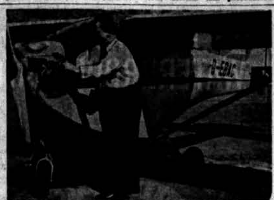
BACK IN THE AIR — First German-made aircraft since the end of World War II is exhibited at the Fifth Annual German Airport Day at Bremen. Called the "Motor-Raub," it's a glider-type plane powered by a Volkswagen engine. It flies for five hours on five gallons of gas.
