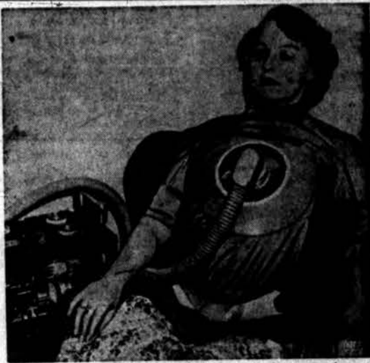
PORTABLE RESPIRATOR —This portable respirator for polio victims is said to be the world's smallest. On display in London, England, the unit consists of the respirator, which is worn like a blouse, and a pump, which may be plugged into an electric outlet or powered by a battery.
