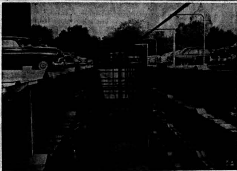
PUSHBUTTON PARKING — Harrisburg, Pa., has one answer to the parking problem — pigeon hole parking. This open air garage is connected to an office building. The elevator slides locked car into space. No hands touch the vehicle. One man operates the whole works with pushbuttons. State capital dome is at right background.
