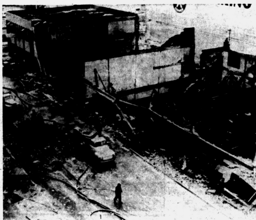
THE AFTERMATH — Firemen huddle around a group of buildings which were wracked by gas explosions yesterday. The store at lower right is where the gas smell was first discovered.
